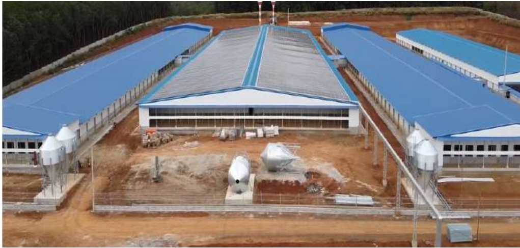
Barns Aerial View
